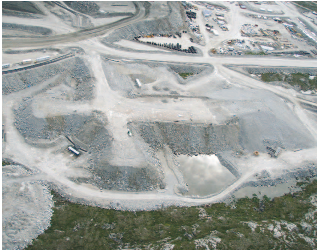
A series of instruments are installed within each test pile to measure temperature water flow, water chemistry, oxygen and carbon dioxide levels, microbiological populations, thermal conductivity, and permeability to air. Outflow from the base of each pile is directed to the instrumentation trailers. The three test piles are to the left, centre bottom and right, with the access ramp (top).
